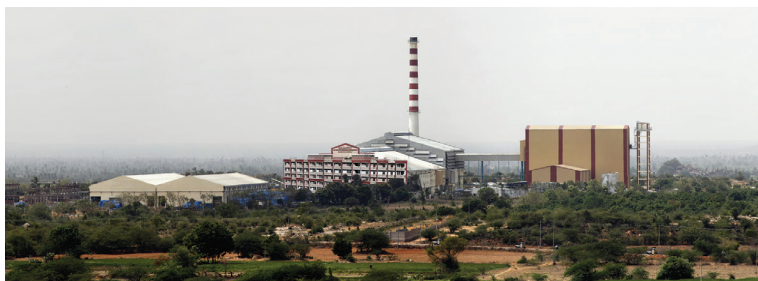
The AGI glaspac glassworks at Bhongir features two melting furnaces, with a combined melting capacity of 1000 tonnes/day
